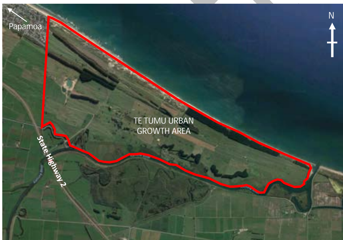
Figure 1.2: Site layout (aerial sourced from Google)
